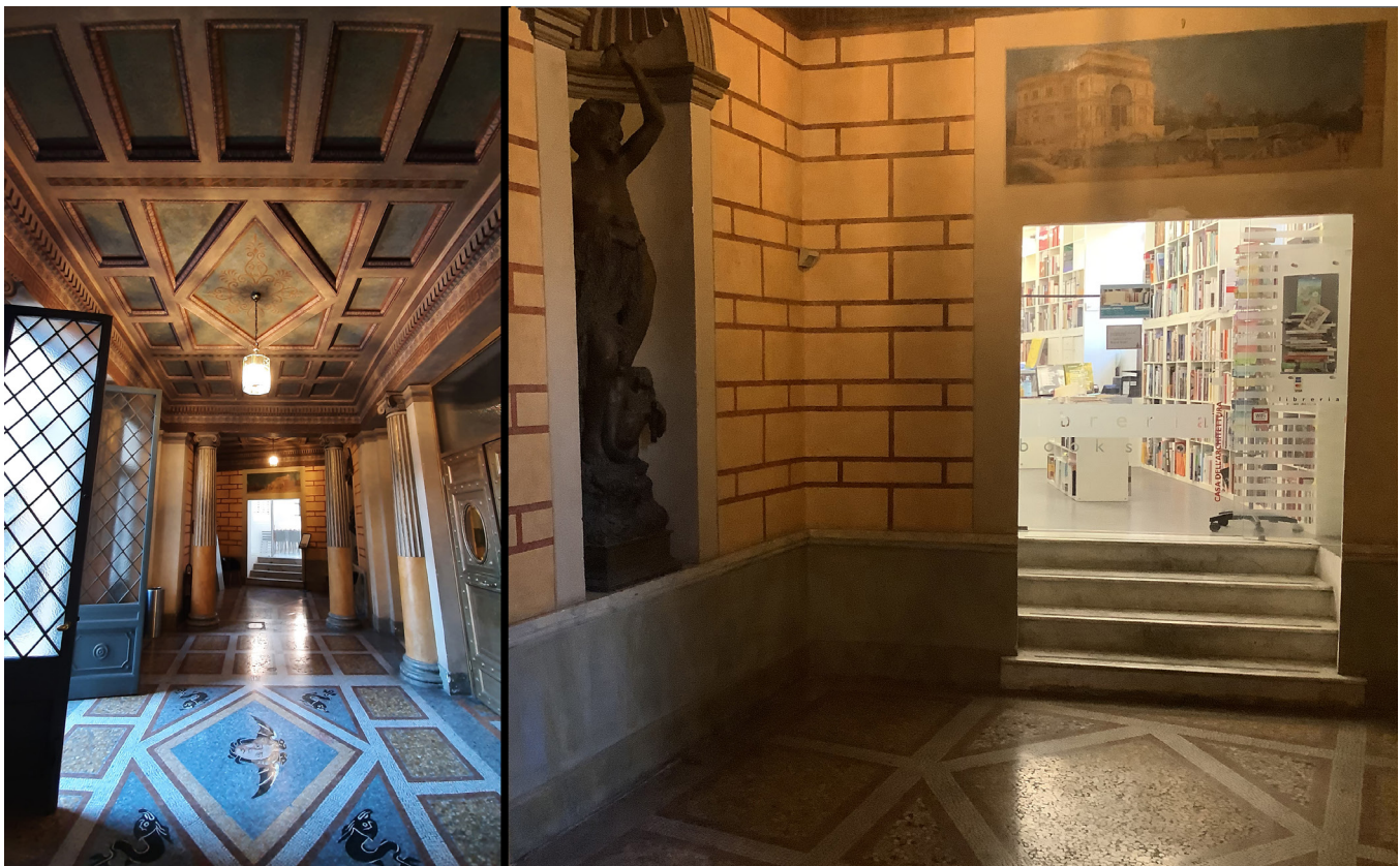
The entrance hall (left), and the right side access to the former technical corridor of the main floor.
