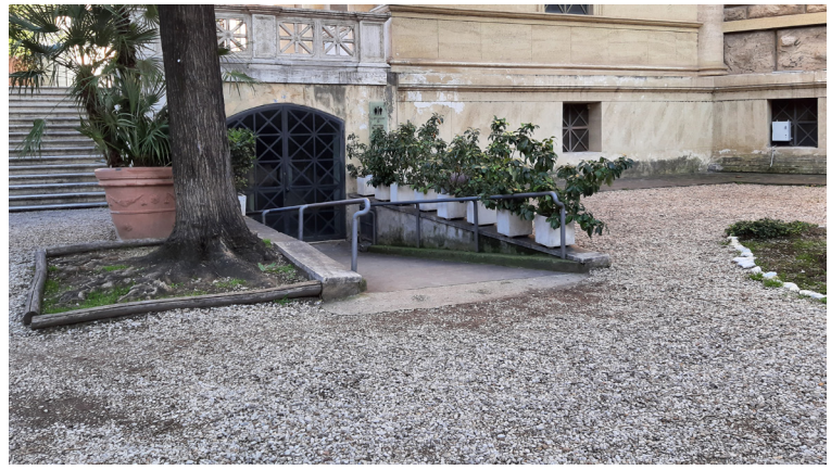
One of the entrances to the basement.
