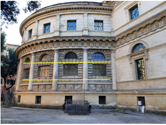
Some of the twenty windows of the former technical corridor. Back then, they were the lighting system of the tanks!
