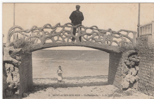
Passerelle (footbridge) on the seaside in Saint-Aubin-sur-Mer, France.
