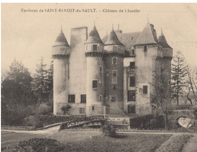
One of the earliest bridges made of reinforced concrete was designed and built by Joseph Monier at the Château de Chazelet, Chazelet, France.
