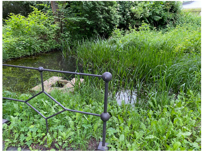
Much of the original technical water management system for the ponds has survived and continues to function to this day.
