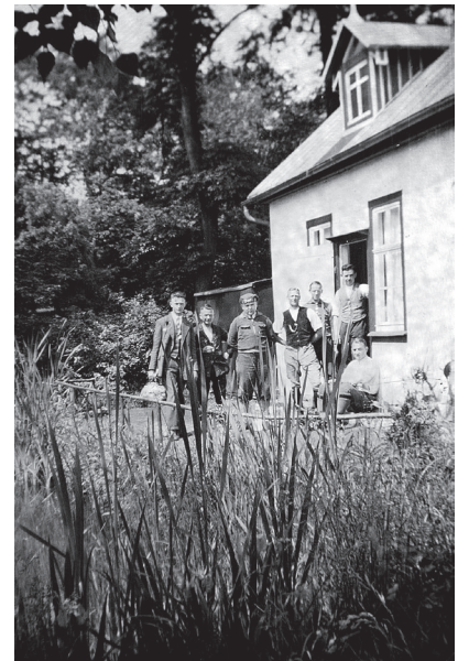
Once plastered and fitted with its extensions, the proud club members could take pleasure in the finished structure.
