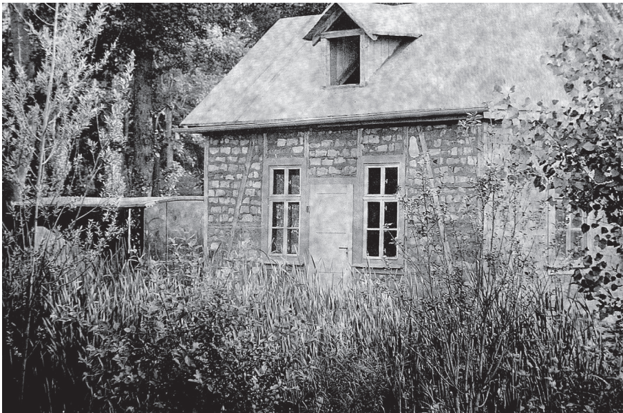
The unplastered shell of the building was completed.
