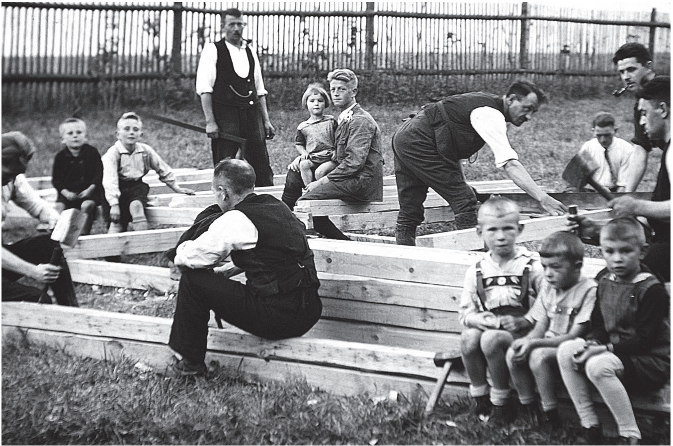
As the final measure, the small clubhouse was erected behind the first pond.
