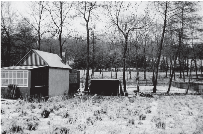
In this winter photograph, the extensions and auxiliary out-buildings are clearly visible from the rear of the clubhouse.
