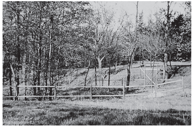
To ensure that the few existing groups of trees were not damaged during construction, they were precautionarily enclosed with temporary fencing.
