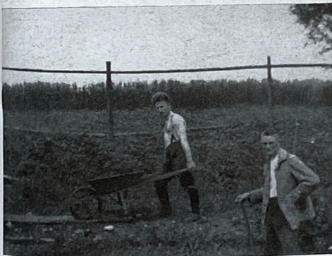
Heavy work, pond 4 is being excavated
