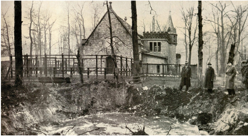
In 1945. Things look bad in the Hannover Zoo! Inspector Eiffert, head gardener Bruns, and his son observe the damage. In the background, the destroyed elephant house.
