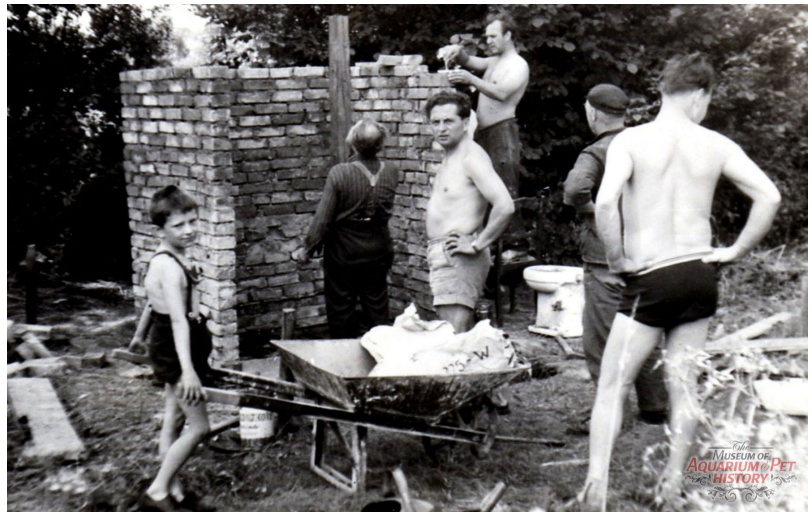
All trades were carried out through voluntary labor; visible here doing masonry work is Friedhelm Amberger, later owner of an aquarium and pet shop in Gotha.
