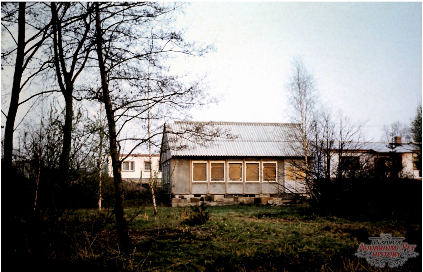
The shell construction is complete.
