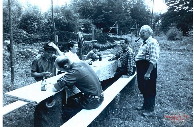
Here, under the direction of Charly Fuchs (right), the foundation for the new barrack-style building is being laid.
