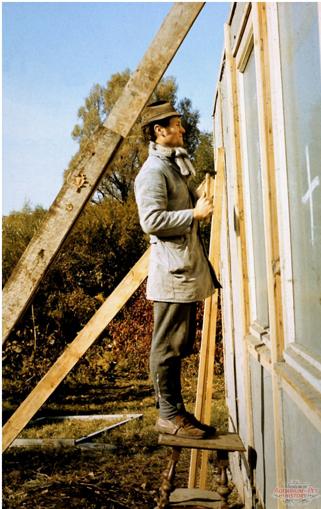
Prefabricated parts are assembled to create the barrack-like structure intended as the future clubhouse.
