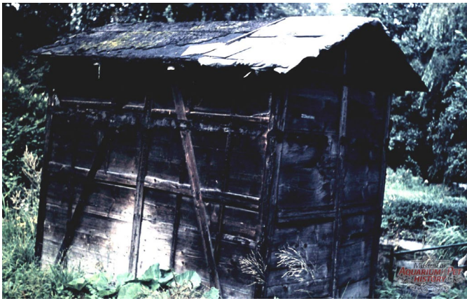
Schaeffer's old wooden hut from 1890 on the island in the Röhrenteich initially still stood.
