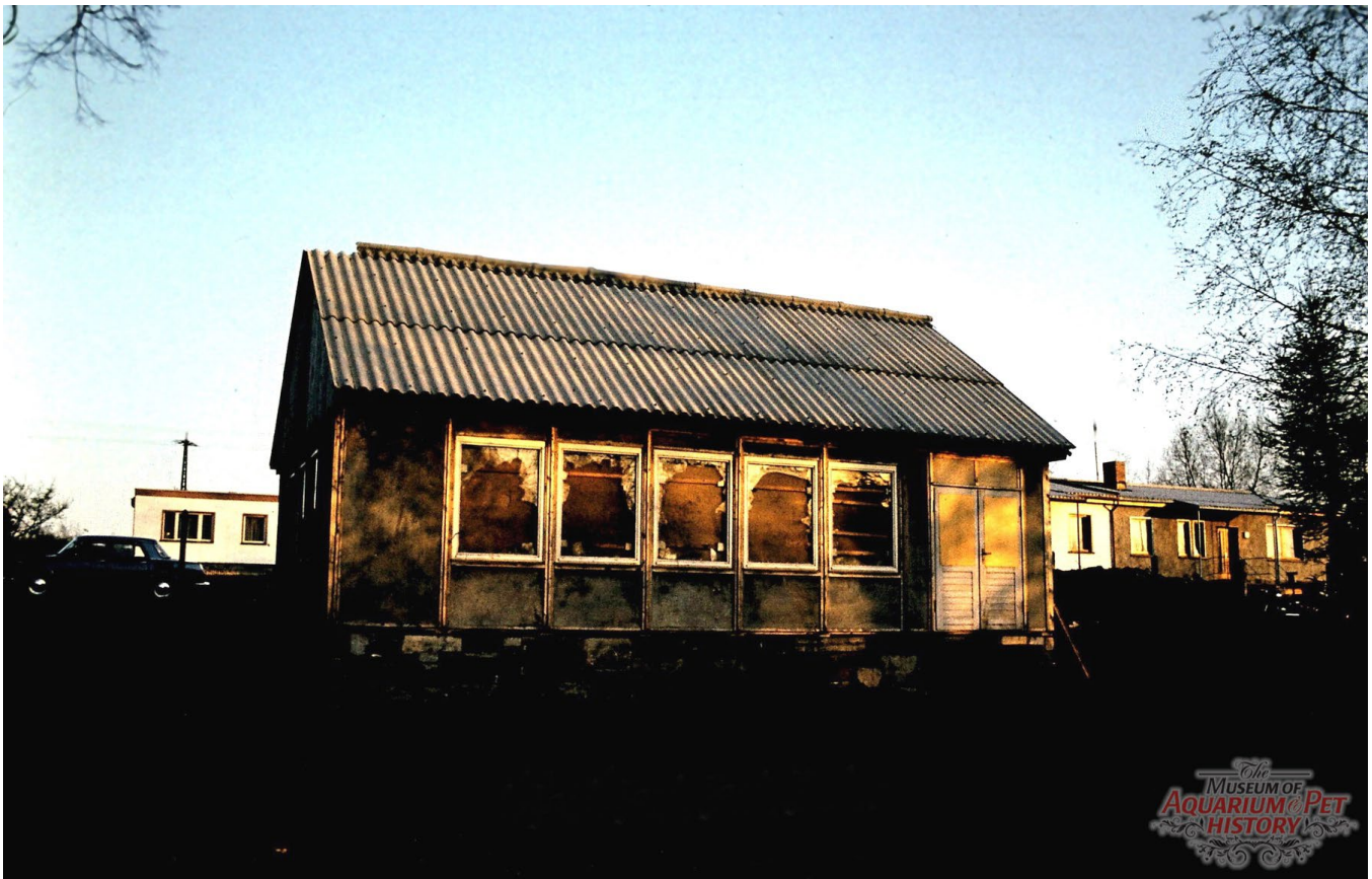
The clubhouse was heavily damaged by vandalism in the 1970s.
