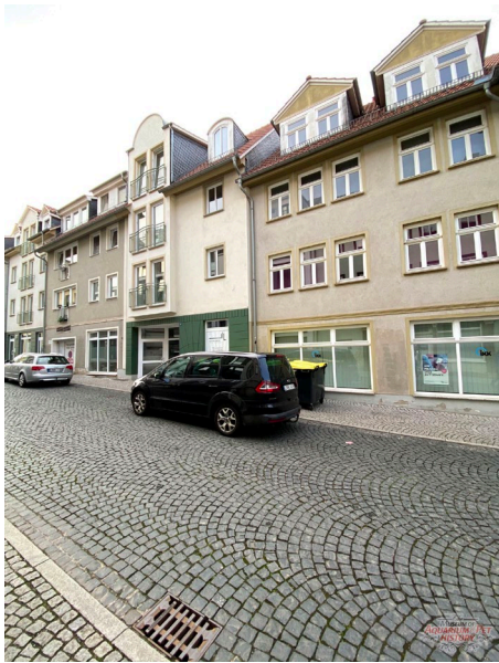
In this building on Gutenbergstraße in Gotha, the pet shop Zoo Kestner was located.
